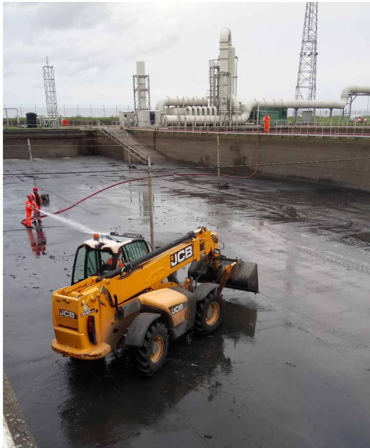
Figure 6.28 Storm tank cleaning operations 5 th September 2017
